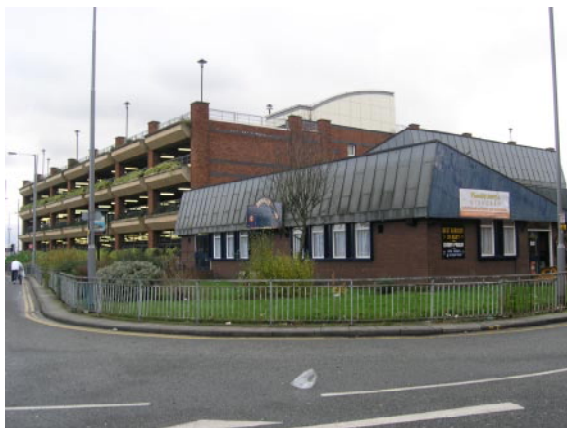
Thwaites PH - largely single storey structure with an opportunity to reconfigure or redevelop as part of an initial or future phase
